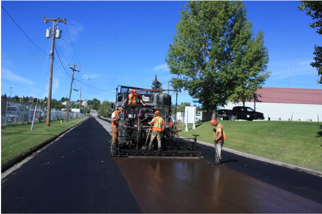
Figure 3. Micro surfacing construction process.
