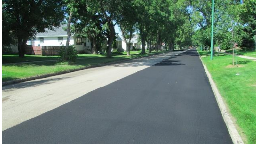
Figure 5. Micro surfacing used in a residential area to preserve pavement condition.
